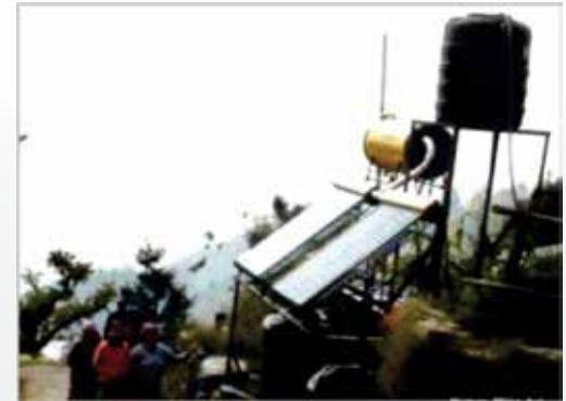
Women filling hot water from Community Solar Water Heater Moolkoti village, Himachal Pradesh
